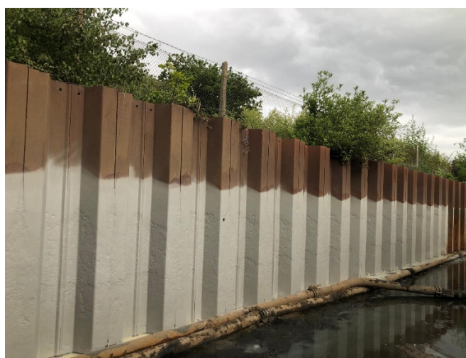
Figure 2: Ultra-high pressure (UHP) water jetting was used to remove corrosion and prepare the steel sheet piles for repair.
