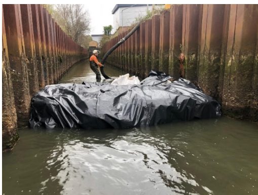
Figure 1: A temporary dam used to create a dry working area.
