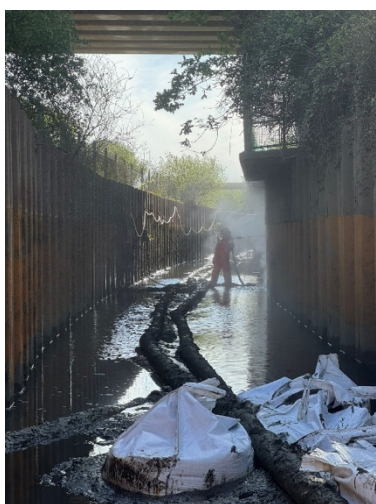
Figure 3: The protective cementitious epoxy coating system being spray-applied to the sheet piles
