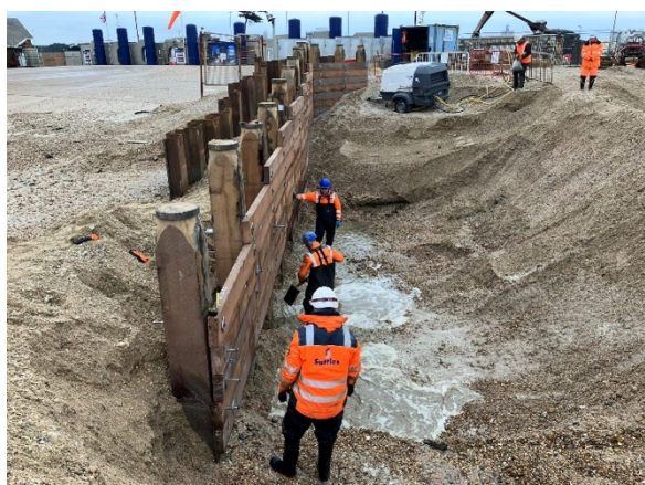
Figure 3&4: Planking
