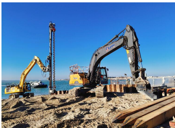
Figure 1&2: Pile installation & Auger Works
