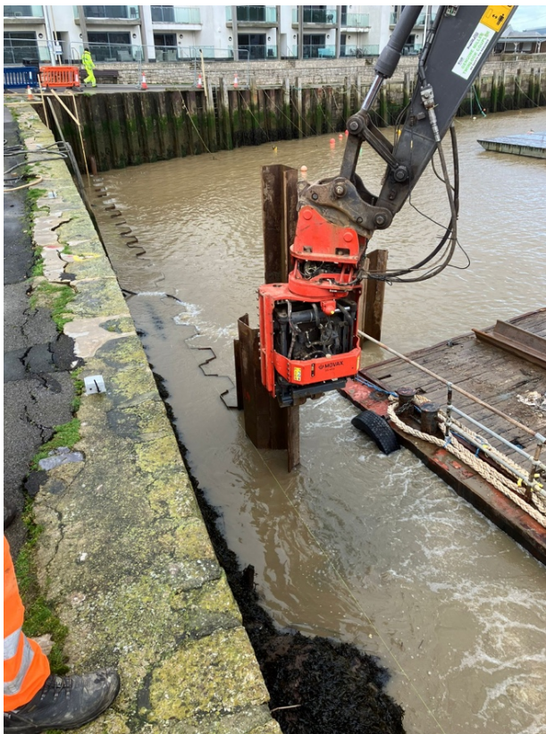
Figure 3: The Movax attachment pushing in the sheet piles
