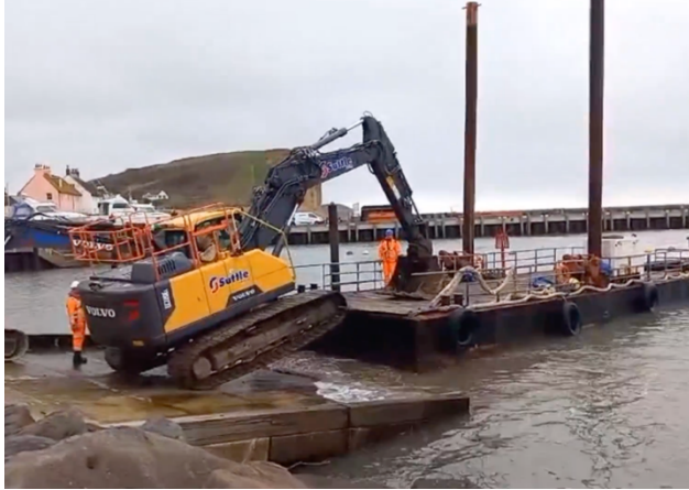
Figure 1: A still taken from footage of the excavator boarding the cargo barge.
