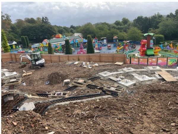
Figure 3: The completed Piles
