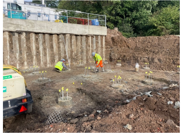
Figure 2: The bearing piles having been installed, filled with concrete and the cages inserted.
