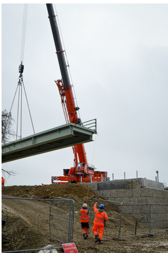
Figure 5&6: The first of the two 21.4m bridge decks being craned into place.
