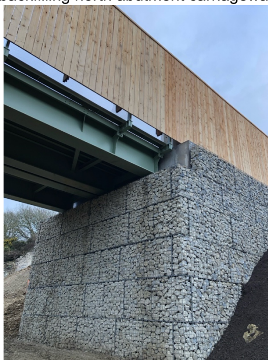
Figure 10: The abutment having been clad in the gabion stone
