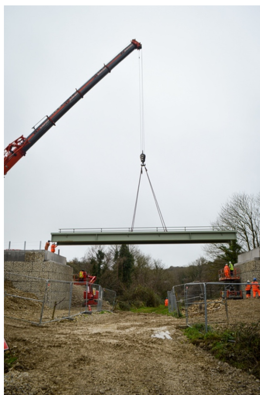
Figure 5&6: The first of the two 21.4m bridge decks being craned into place.
