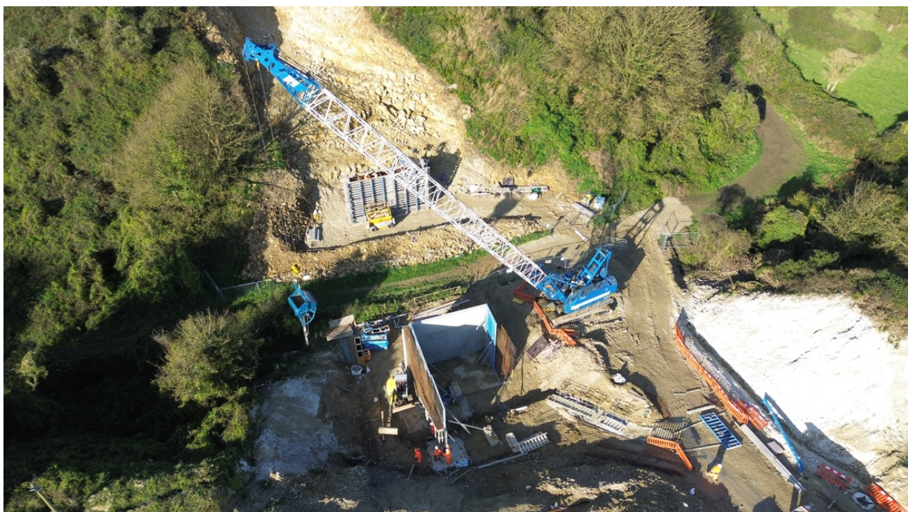
Figure 1: A drone view of the formwork being cast for the bridge abutments.
