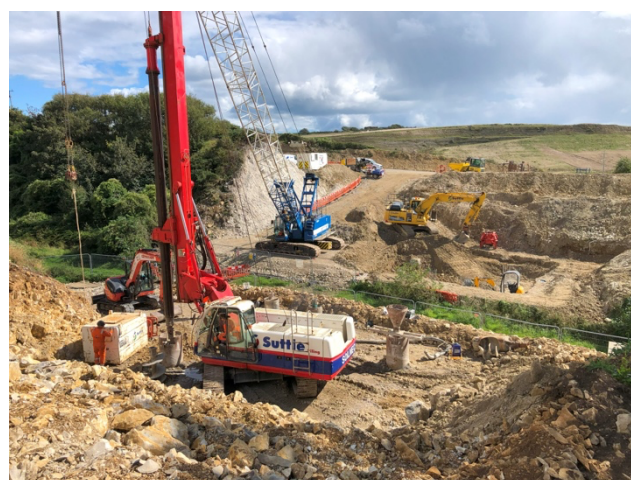
Figure 3: Rotary bored piling works.
