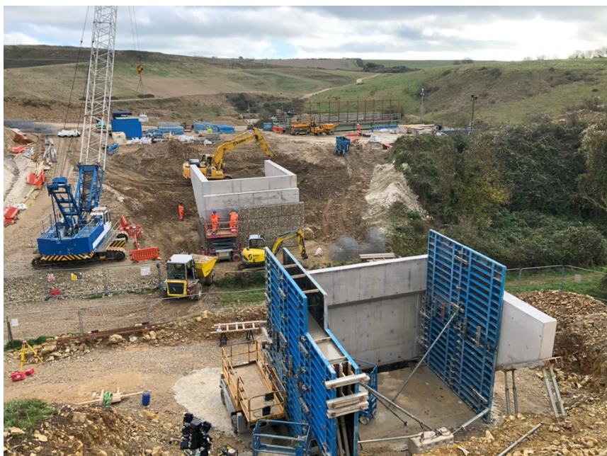
Figure 4: Reinforced concrete abutments and gabion cladding.
