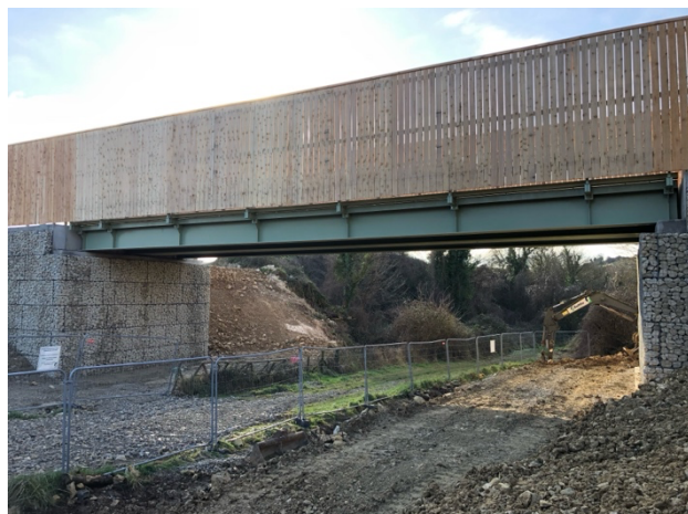
Figure 7&8: Installation of timber cladding and backfilling north abutment carriageway.
