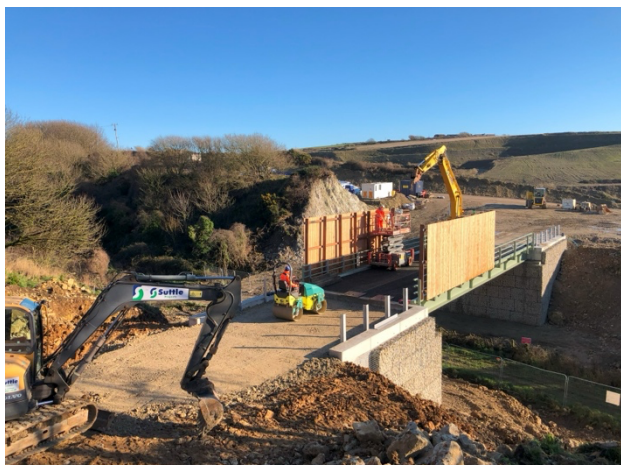
Figure 7&8: Installation of timber cladding and backfilling north abutment carriageway.
