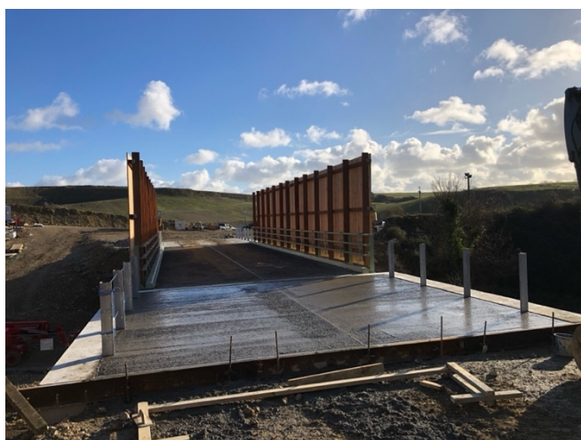
Figure 7&8: Installation of timber cladding and backfilling north abutment carriageway.
