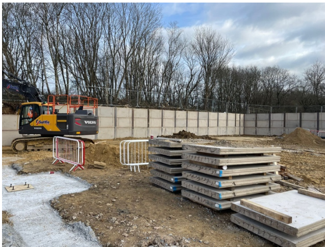
Figure 1: The site with part of the kingpost wall
